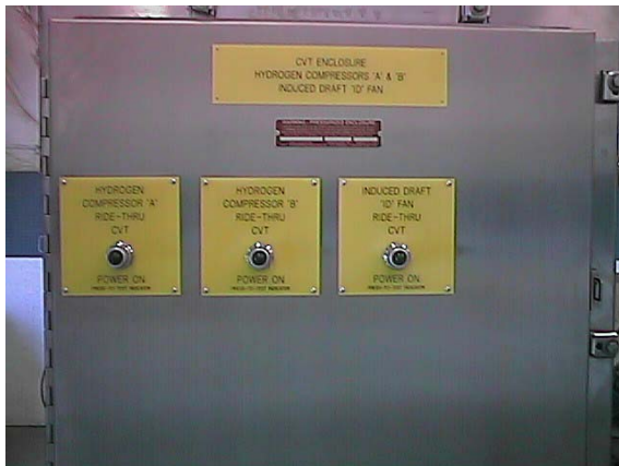
Figure 5. CVT enclosure front panel tags for two hydrogen compressors and one induced draft fan ride-through systems.
